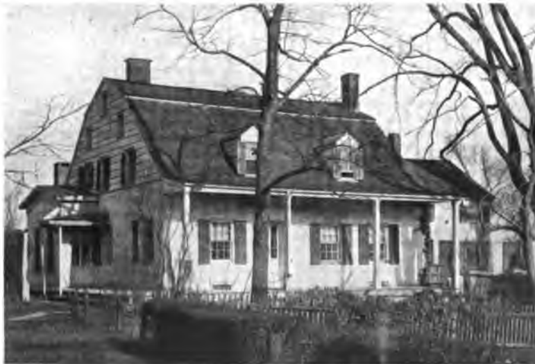
THE DUTCH COLONIAL GAMBREL-ROOFED TYPE A typical Dutch Colonial house, the Terhune homestead, at Hackensack, New Jersey (The dormer windows in the roof are a later addition)
